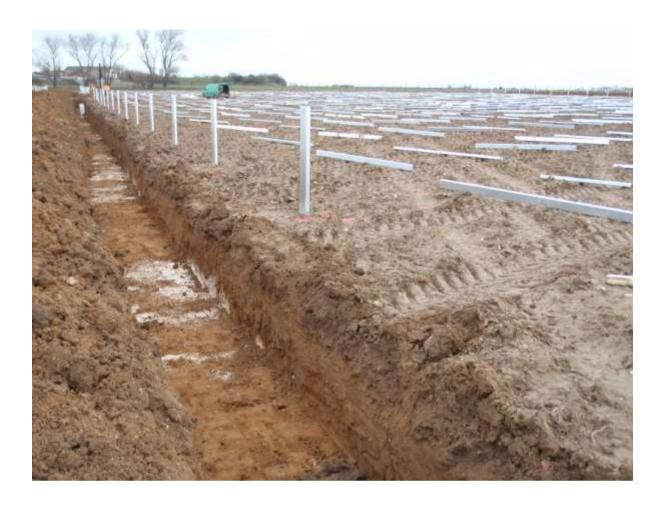
Plate 4. Main cable runs excavated with ditching bucket (looking north)
