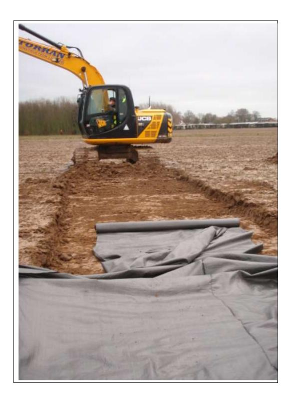
Plate 2. Access road construction with ditching bucket (looking east)
